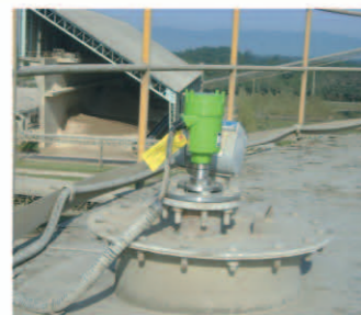
Radar Level Transmitter for Cement silo
