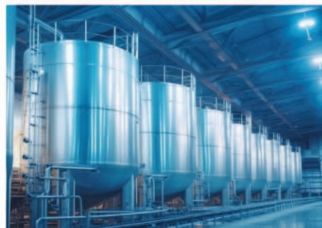
Liquid level control in tanks and pits (Pump control, upper and lower limit alarm)
