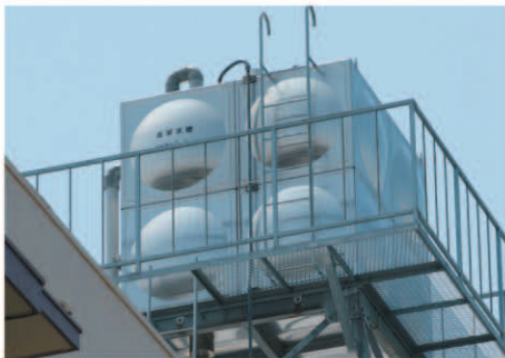
Water tank, Elevated water tank
